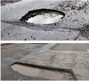
Fig. 7. Example of potholes.
